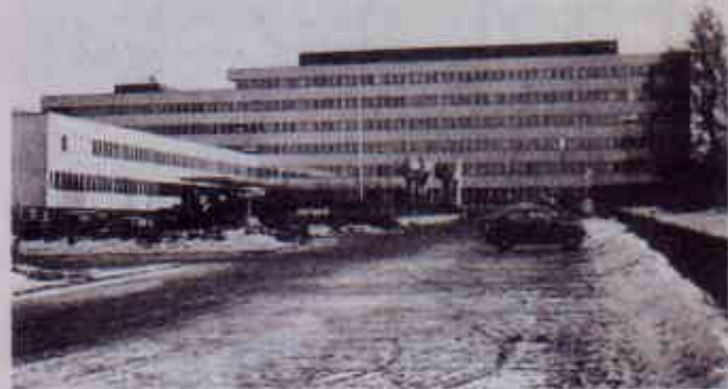
Central Hospital, Lahti, Finland. VAV system uses four Varofoil fans.
